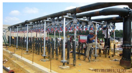
PBHS Valve House Piping - During Construction
