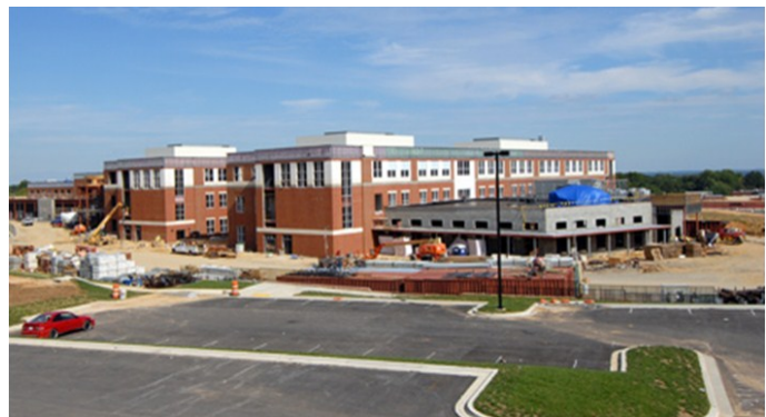
PBHS BUILDING UNDER CONSTRUCTION—LEED GOLD
