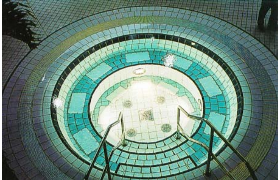
Photo from above a built-up whirlpool. The jets are switched off for the photo. The plates in the seat and floor allow an even flow of air upwards. The entire whirlpool offers jet action, not limited to individual nozzles. There is a 100% over the rim gutter system to wash away impurities from the surface. This results in significantly cleaner water than whirlpools using skimmers.
